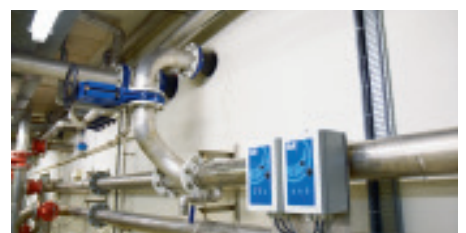
After fermentation, sludge is transported to a sludge buffer storage before final dewatering.
