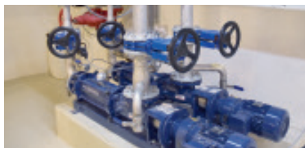
Sludge from the bottom of the clarification zone in the DEMON® tank is pumped back to the process as return sludge, and excess sludge is pumped into a cyclone, where anammox bacteria are sifted out.
