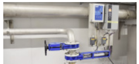
AVK knife gate valves with linear actuators on a reject water pipeline. The linear actuators were chosen, since they are energy efficient compared to actuators using compressed air
